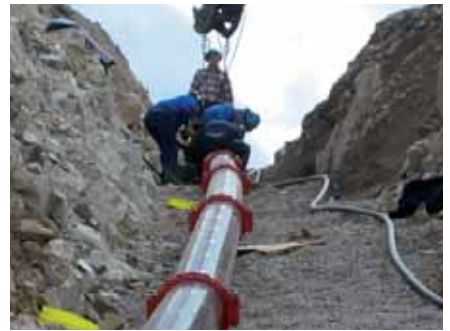
Installation of pipes for water supply to the snow guns. Idrefjäll Sweden.
