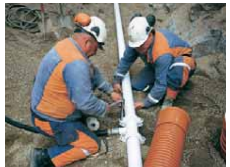
The city of Lidingö, Sweden, uses the Alvenius® thermoplastic coated pipe system for distribution of potable water.
