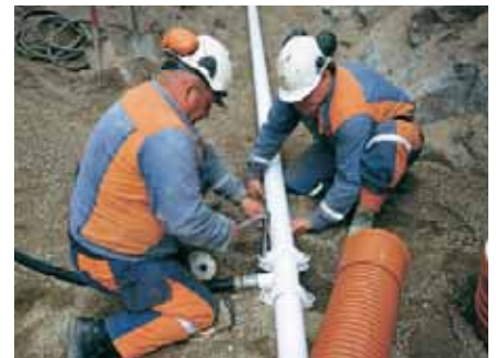
The city of Lidingö, Sweden, uses the Alvenius® thermoplastic coated pipe system for distribution of potable water.
